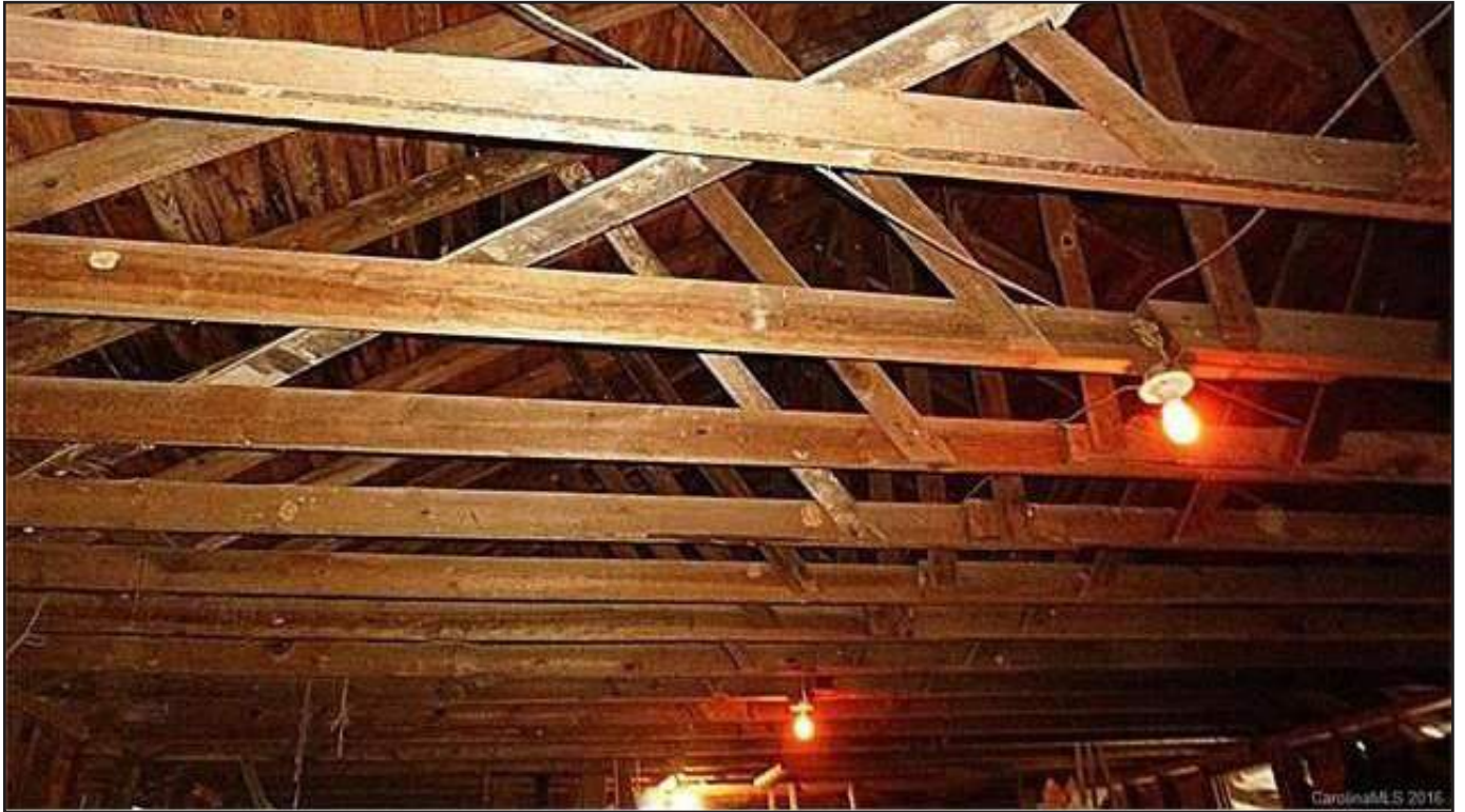
Photograph 11: Interior of mill, ceiling rafters. Source: Carolina MLS, 2016. ( https://www.zillow.com/homedetails/717-Howards-Creek-Mill-Rd-Vale-NC-28168/2103284418_zpid/ )
