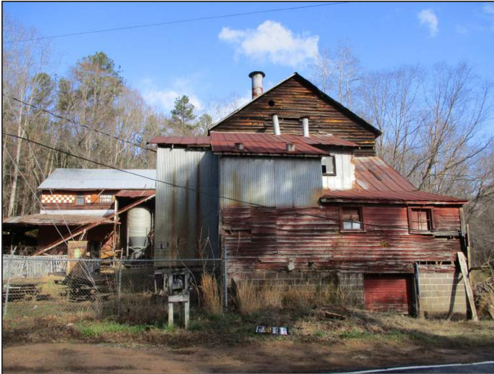
Photograph 3: Facade (south elevation) of Howard's Creek Mill; looking north. (2017)
