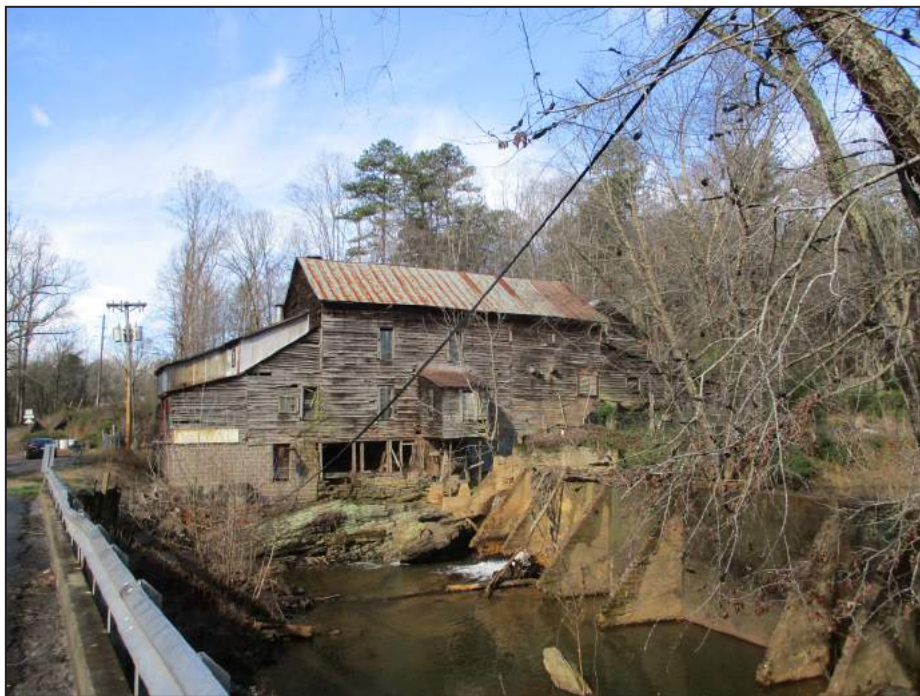
Photograph 1: East elevation of Howard's Creek Mill; looking west. (2017)
