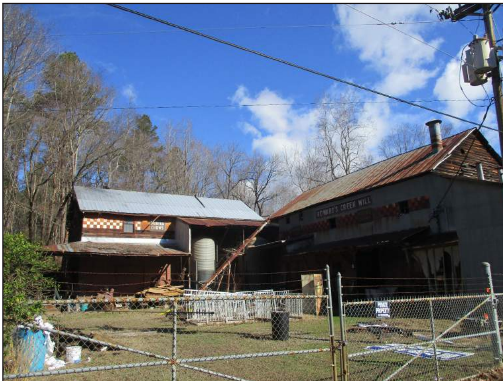
Photograph 7: West elevation of mill and south elevation of ell addition; looking northeast. (2017)
