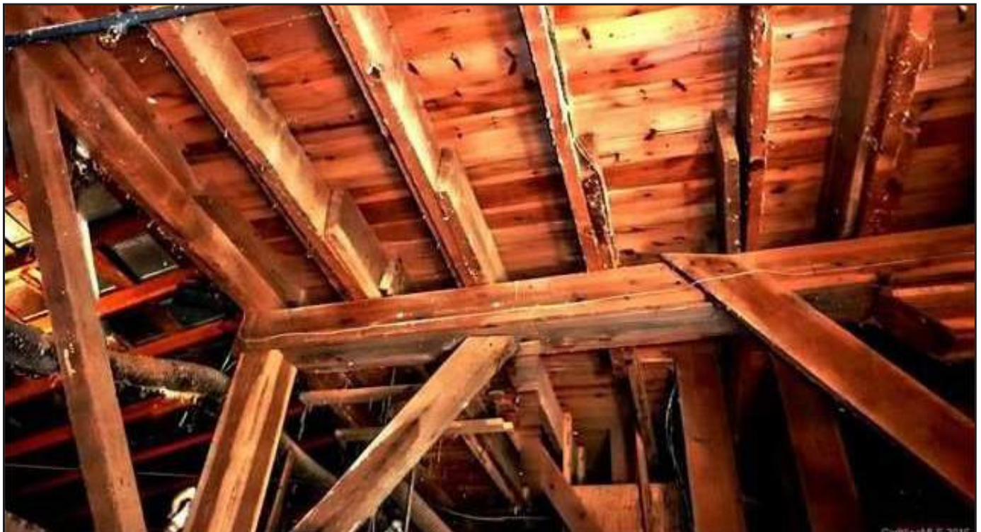
Photograph 12: Interior of mill, ceiling rafters. Source: Carolina MLS, 2016. ( https://www.zillow.com/homedetails/717-Howards-Creek-Mill-Rd-Vale-NC-28168/2103284418_zpid/ )
