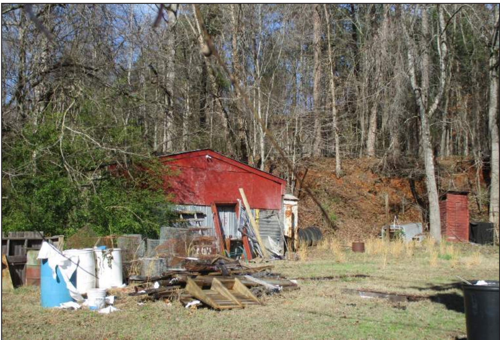
Photograph 10: Large one-story shed, c. 1930; looking northwest (2017)
